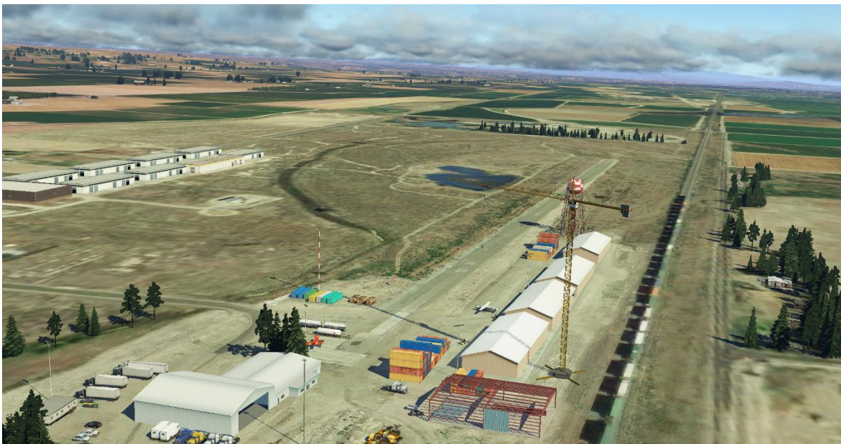
Seen from South
